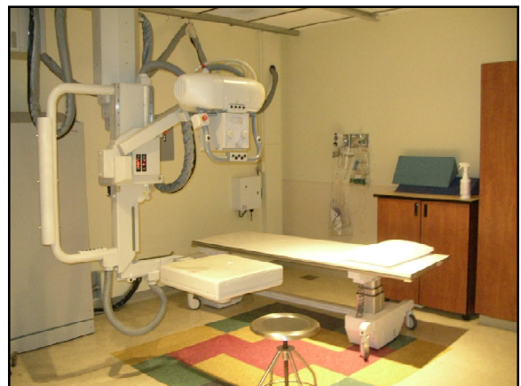
Renovation of Emergency Room Radiology
